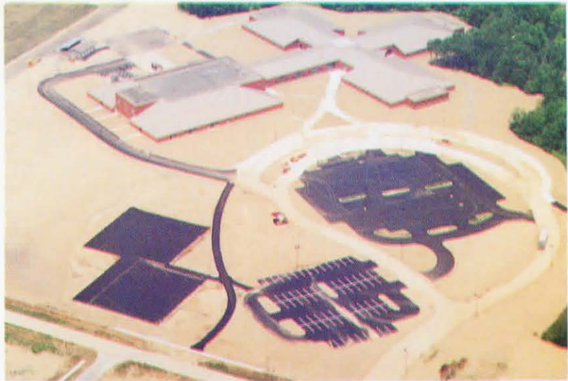
An aerial view of the nearly completed structure.
