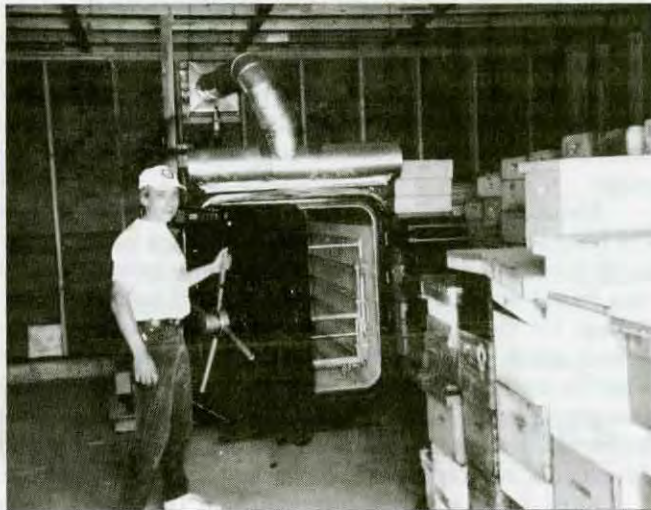
The fumigation chamber is almost ready to operate.
