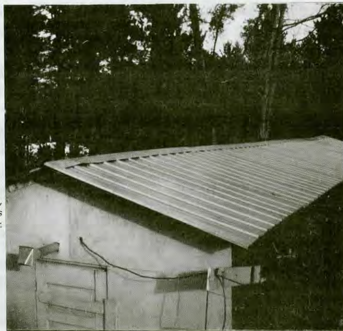
The South end, showing roof, vents and human door.
