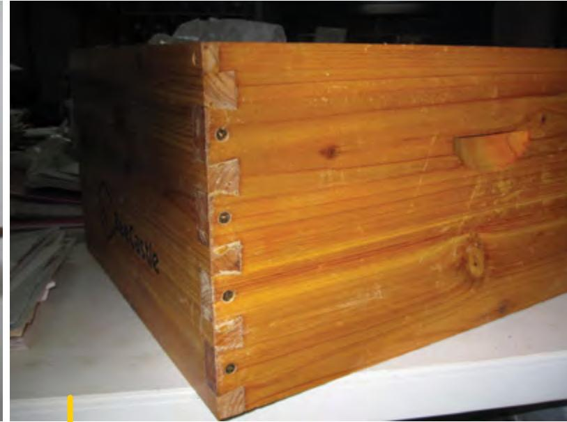
*(Figure 4) Through Dovetails*
