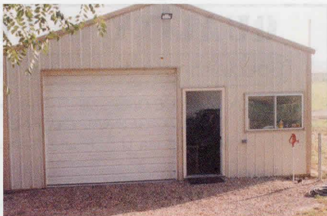
Entrance to honey house building dimensions, 26 x 35 ft. Left side, Loading & storage, right, honey processing.
