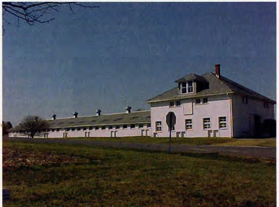
Our current storage barn. The wing was to be demolished.
