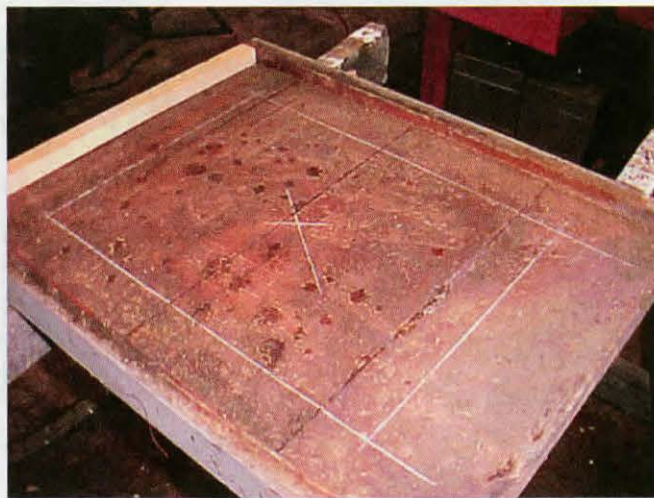
Reference lines ready for hole boring and subsequent cutting.
