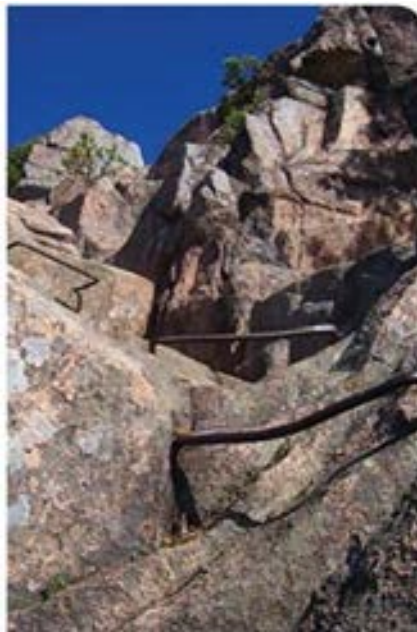
Some of the iron rungs on a trail going up the Beehive.
